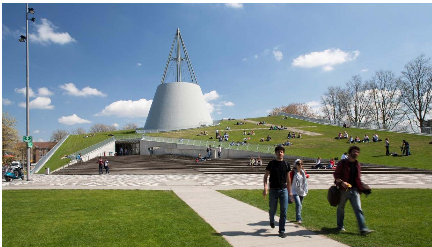
Delft University of Technology Library: grass roof and central steel cone bringing daylight into the central Library space 157
